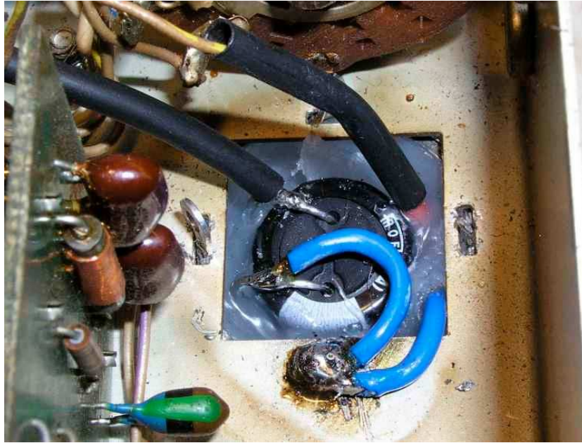
Picture 11: Restored cap in place
